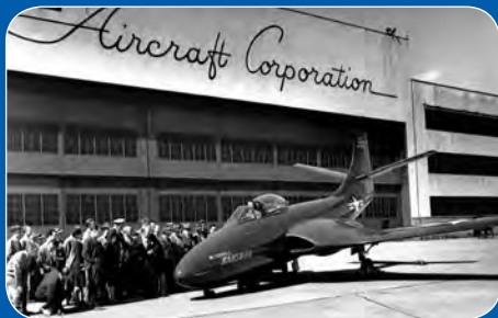
PHOTO: At a 1947 press conference, a McDonnell test pilot engages the outward-folding landing gear causing the XF2D-1 Banshee to take a bow. BOEING ARCHIVES
