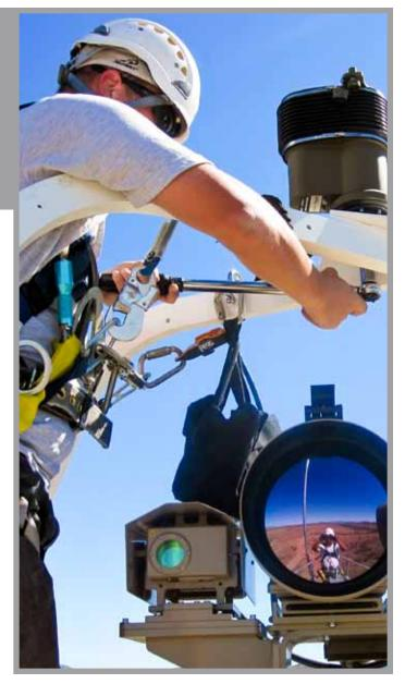
training, Peck can only access the top of the tower via a bucket lift but still dresses in a full harness, hooking to an anchor point on the bucket. Once he safely makes the transfer from the bucket and hooks his lanyard to the platform, he begins verifying that all the tower's radio and sensor connections have been completed correctly by program subcontractors.
