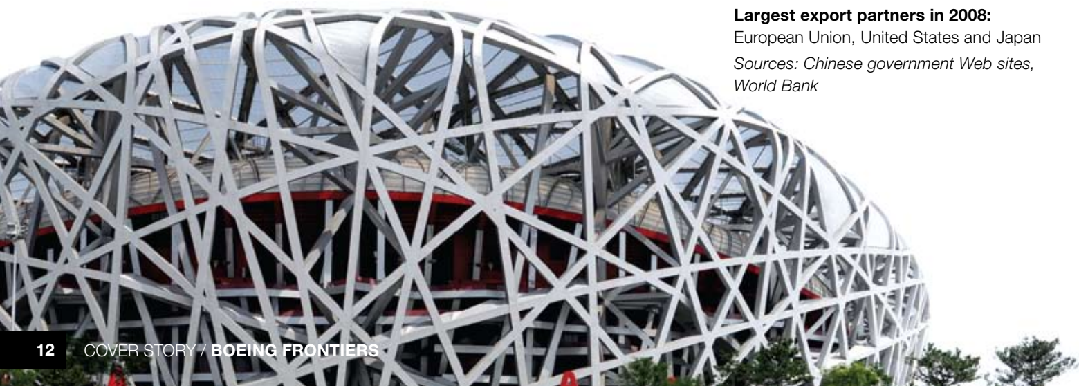
PHOTO: (BELOW) China’s Beijing National Stadium was built for the 2008 Summer Olympics. It was nicknamed the Bird’s Nest because of the structure of steel beams. SHUTTERSTOCK.COM
