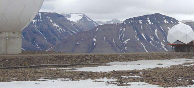
Last summer, a team from Satellite Operations and Ground Systems at Integrated Defense Systems installed and integrated a new Iridium Satellite Telemetry Tracking and Control ground station in far northern Norway. Here, an antenna radome is transported to the Earth Terminal site. The radomes had to be constructed in a protected area to avoid being damaged by high winds.
